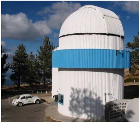
Figure 3.2: 0.84m telescope building
